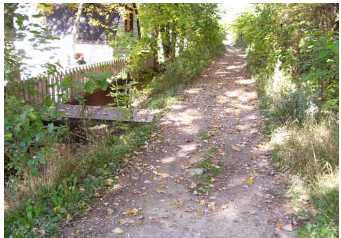
Figure 18 – Overgrowth on Flanking Dike
