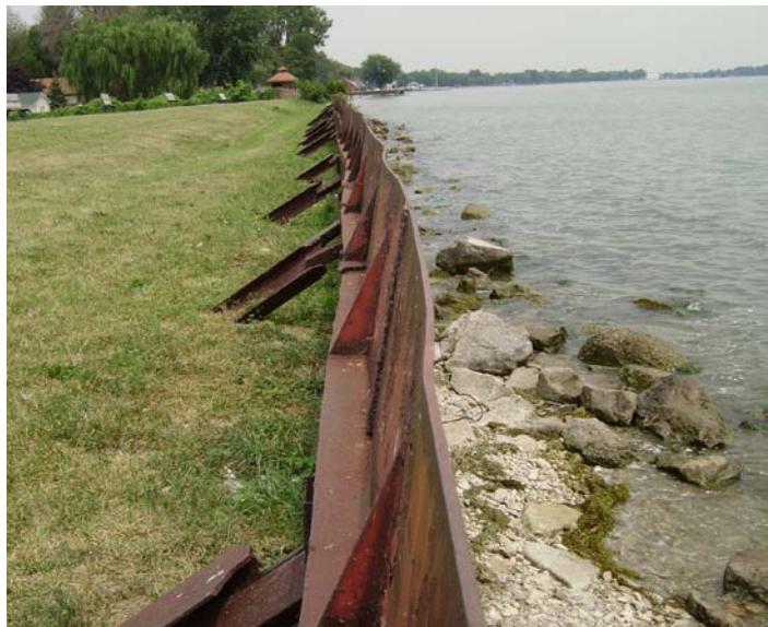
Figure 3 – Temporary Steel Wall
