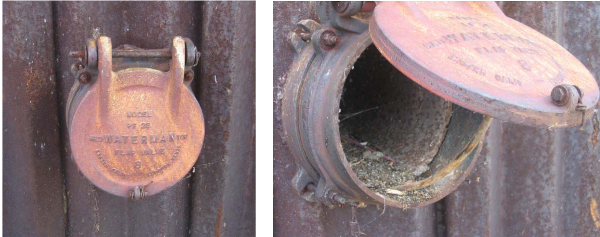
Figure 19 – Flap Gates - Flap Gates cover drainage tubes to dewater catchment areas behind SSP walls.
