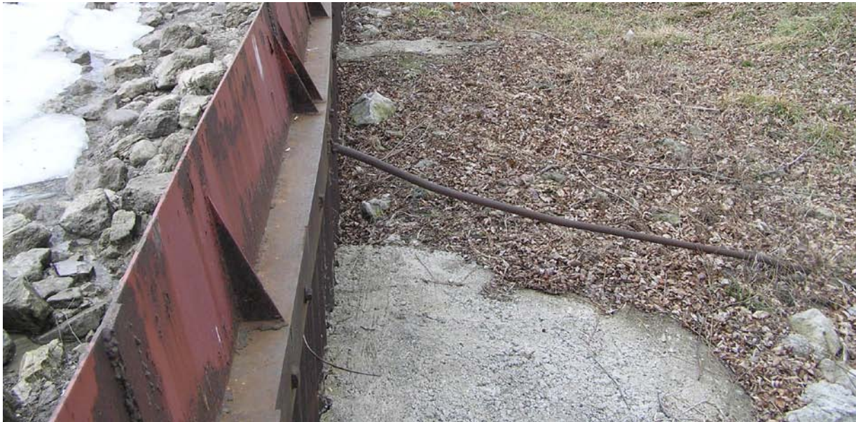
Figure 16 – Exposed Tie-Backs - This tie-back has been exposed due to washout behind the flood protection structure.
