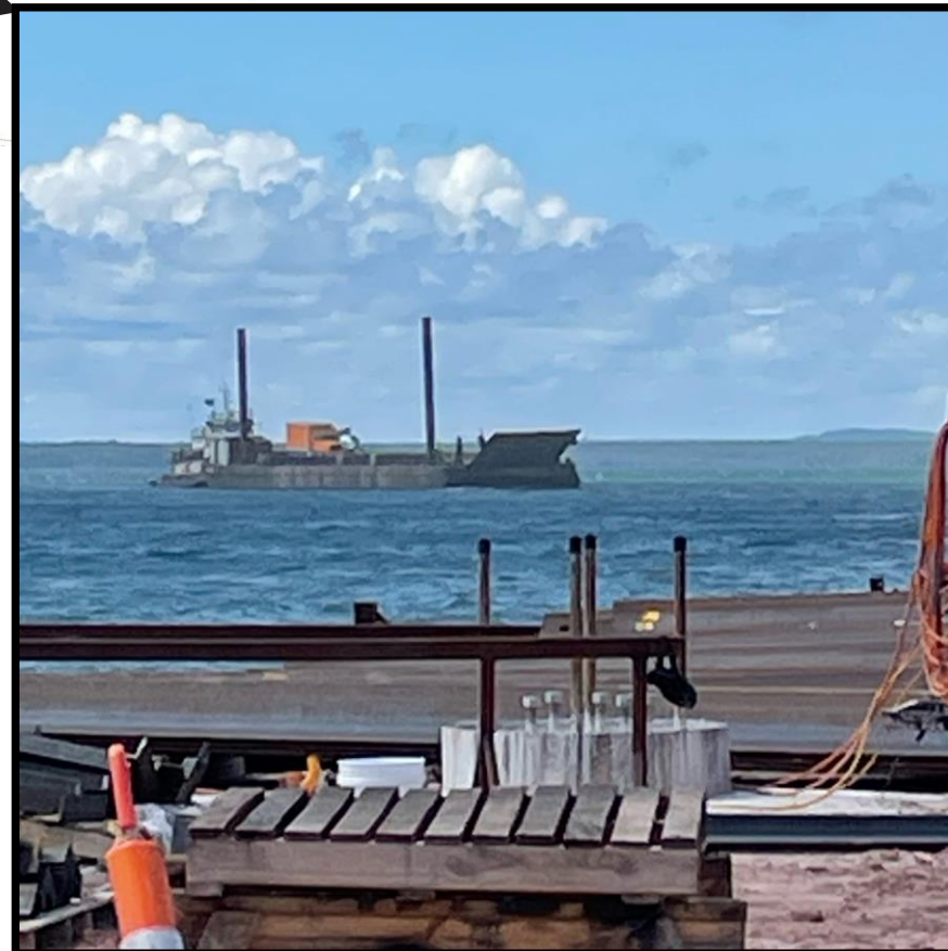
Lubrication truck crossing navigation channel to access construction site
