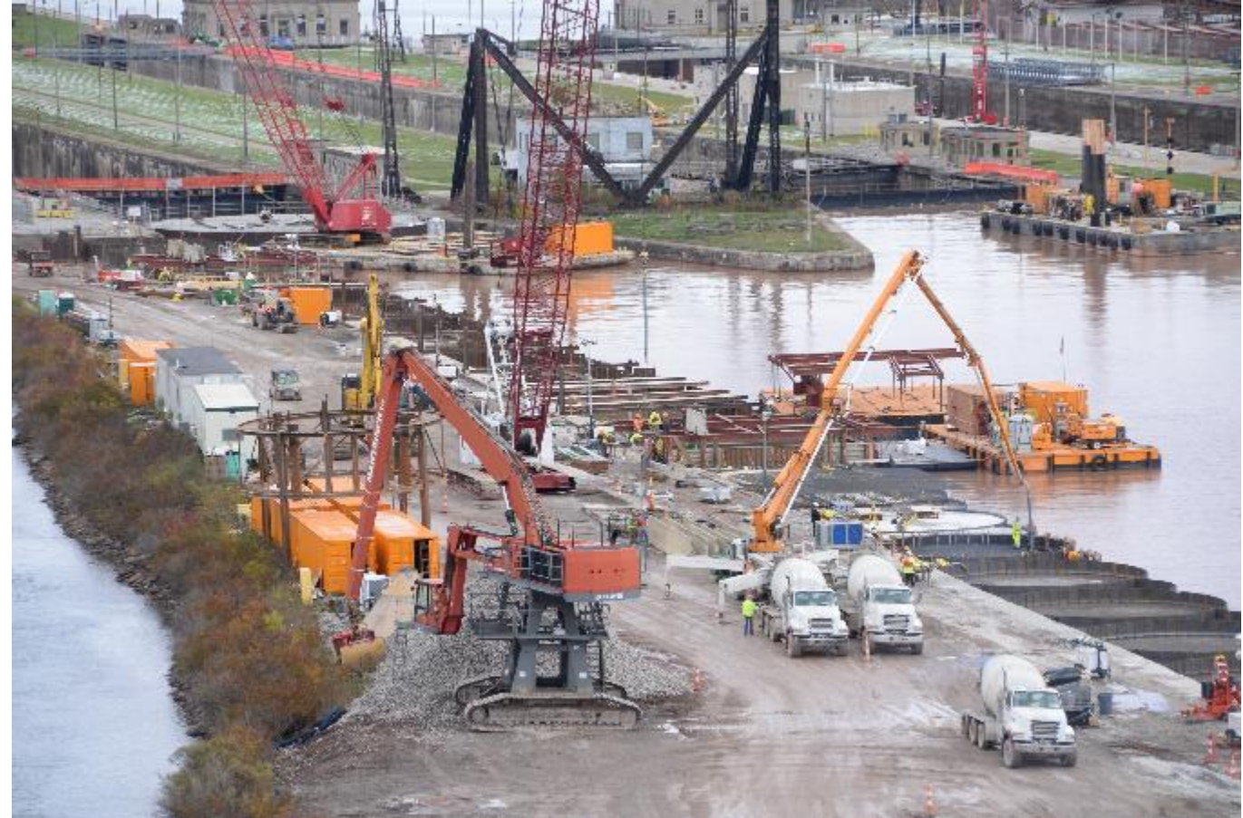
Upstream Approach Wall Tremie Concrete Placement
