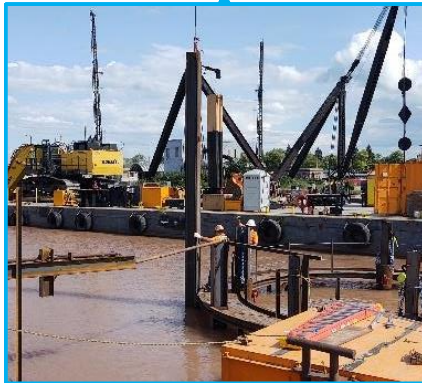
Sheet piles are 30' strips of steel placed within coffer cell template
