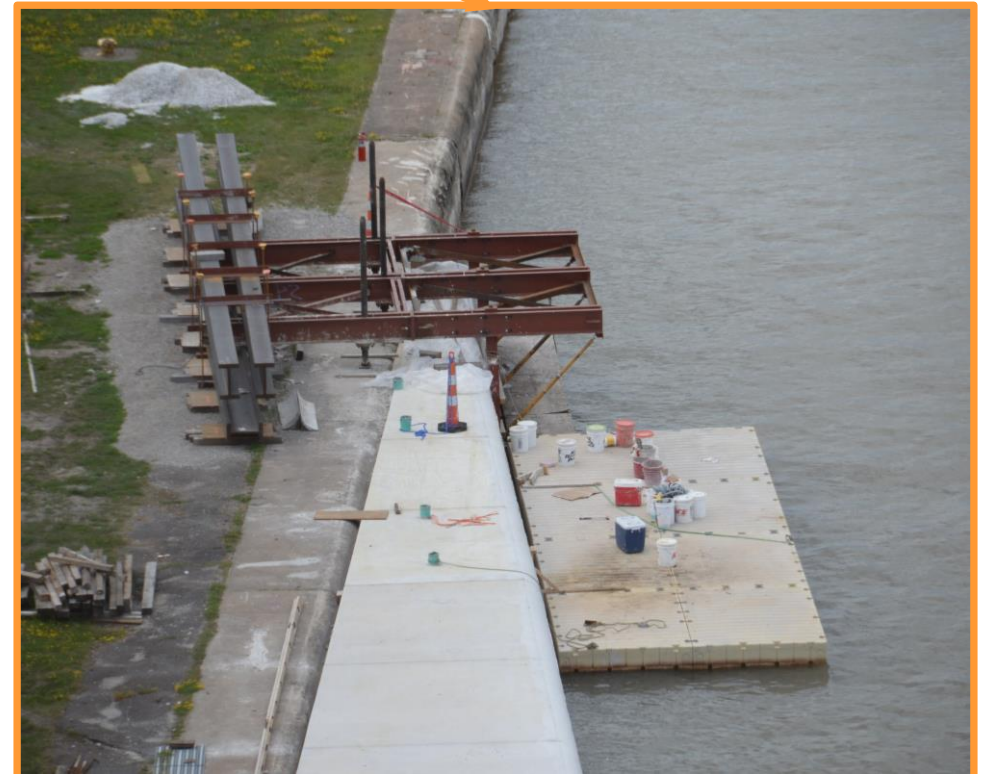
Southwest SSP transition wall with concrete cap
