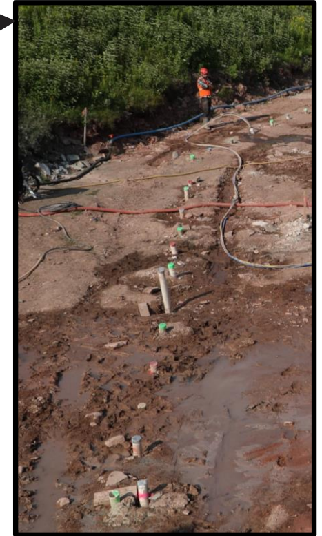
Grout curtain installation
