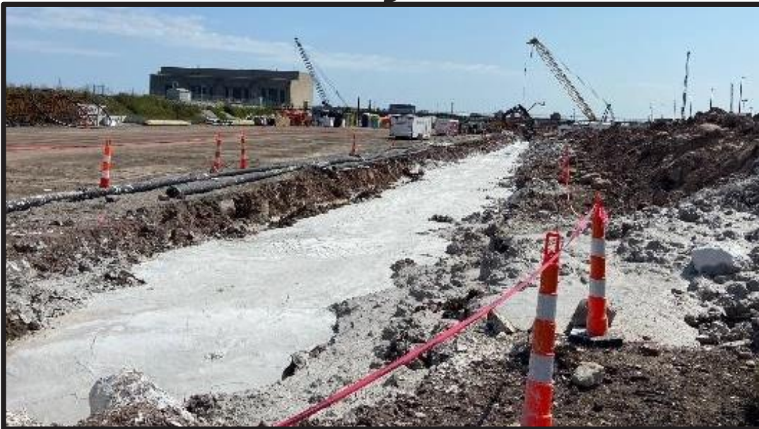
Placement of the Soil Cement – Cement Bentonite (SCCB) wall north of the Sabin Lock to prevent seepage through soil into the dewatered excavation area
