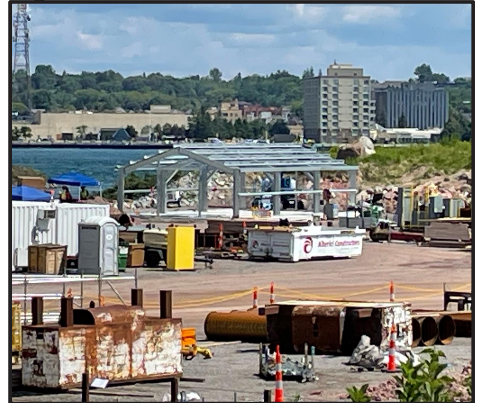
Construction of temporary rock core storage building
