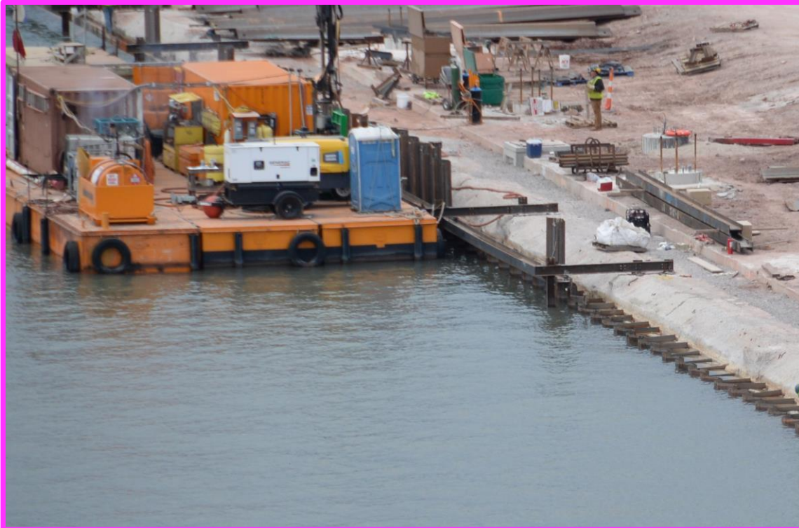
Placement of SSP for SSP faced wall
