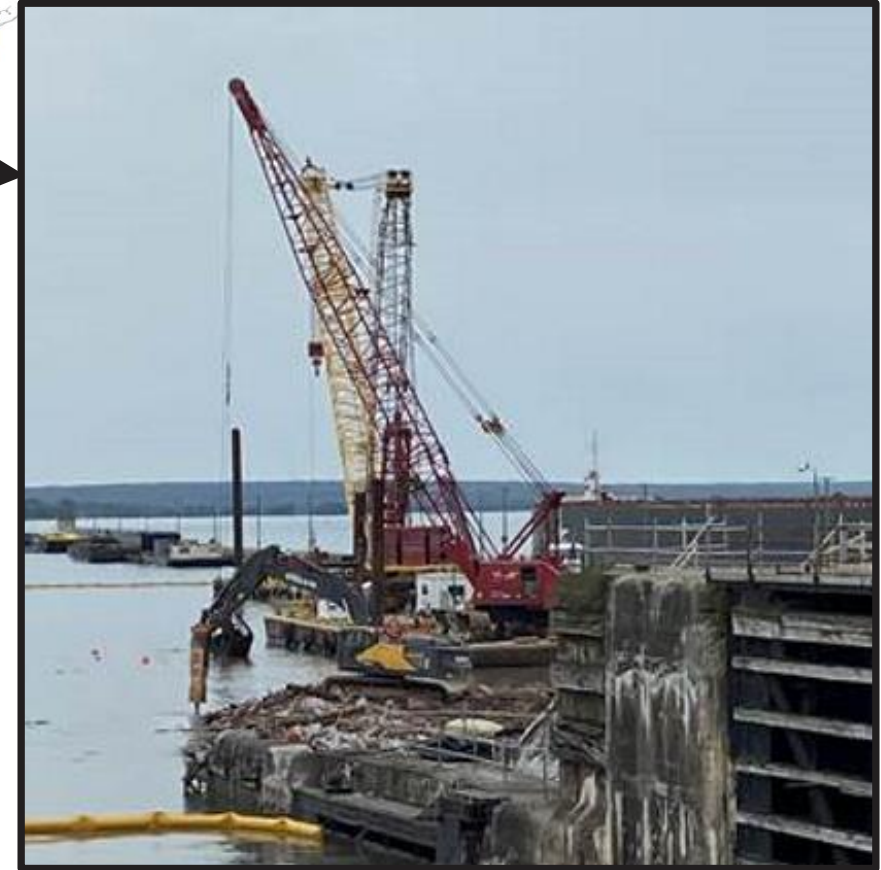
Demo of downstream nose pier in preparation for downstream cofferdam construction
