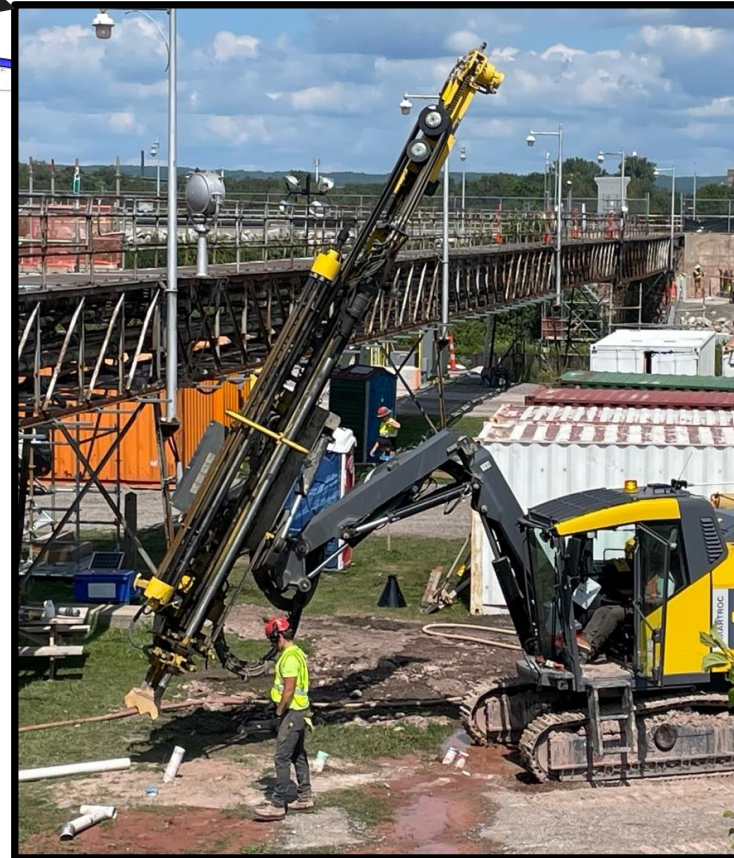
Drilling of shafts for grouting
