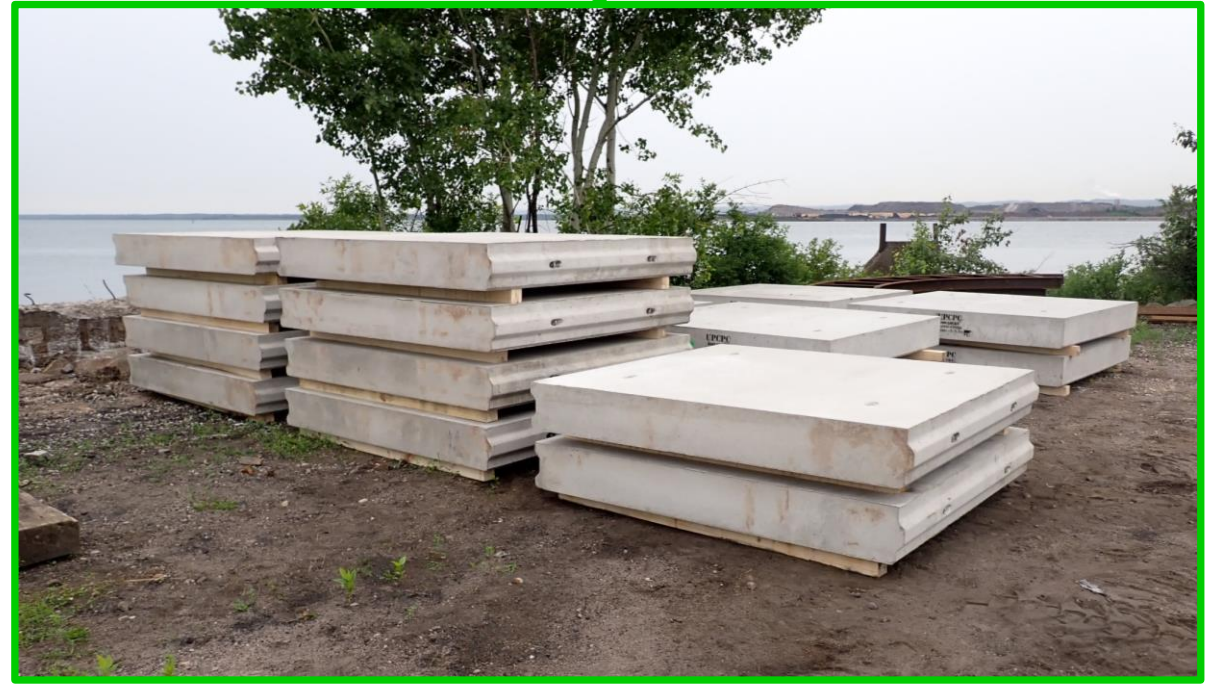
Concrete panels for H-pile and concrete panel wall
