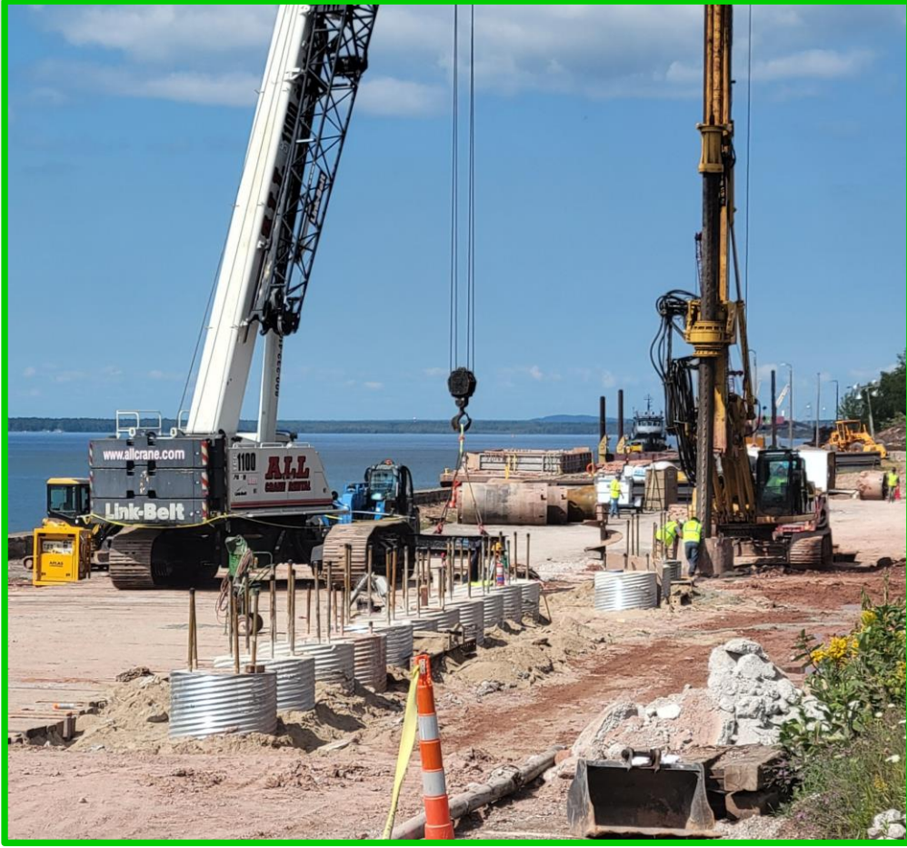
Drilled shaft installation of concrete panel deadmen
