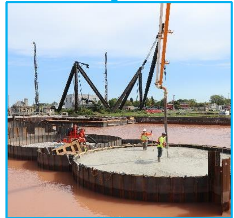
Concrete placement in cell
