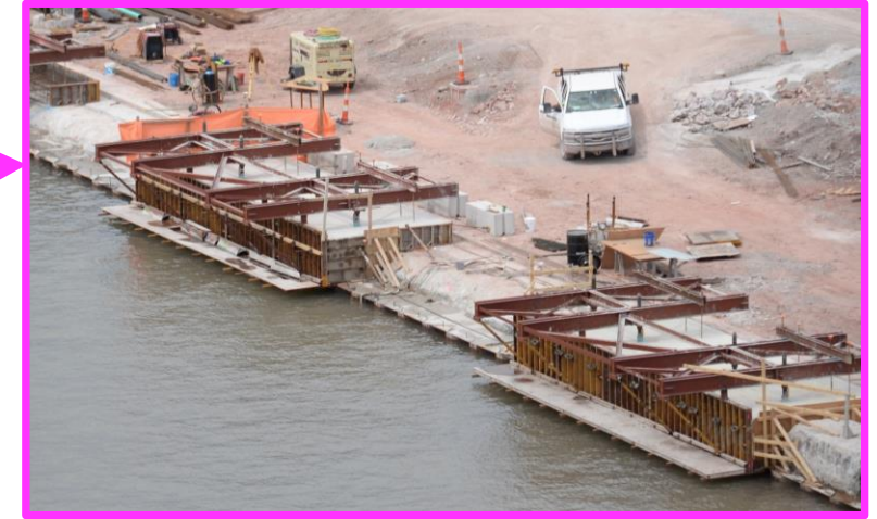
Formwork for concrete caps on SSP faced wall
