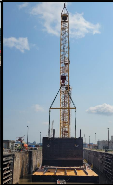
Davis Lock upstream miter gate leaf removal
