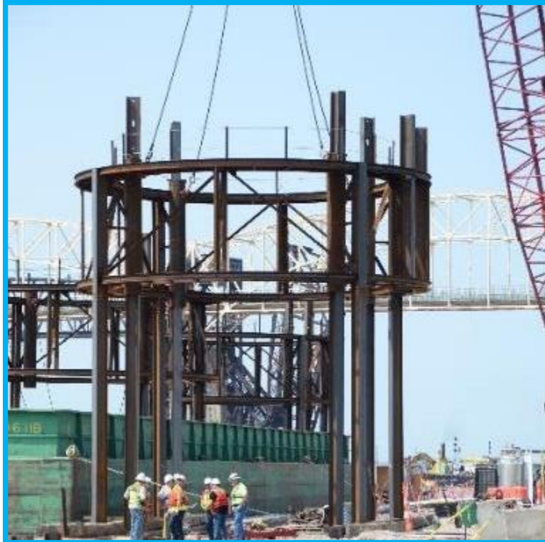
Template used to construct circular steel sheet pile cells
