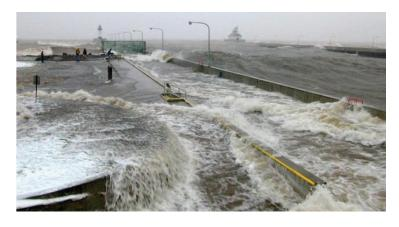
The photo above (*Duluth-Superior Harbor*) depicts large waves engulfing a harbor entrance. In addition, massive ice floes can literally engulf breakwaters (*below – Petoskey Harbor, MI*). The top of the breakwater is barely visible in the ice. Coastal structures constantly exposed to these forces year after year gradually weaken, which can eventually lead to partial or total failure of the structure if adequate maintenance is not performed.
