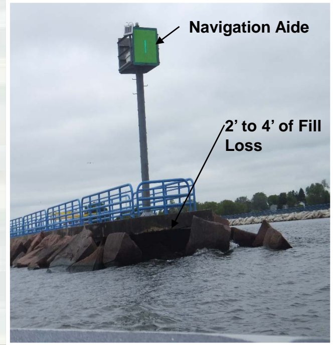
Two Rivers, WI – Ice damage to south breakwater
