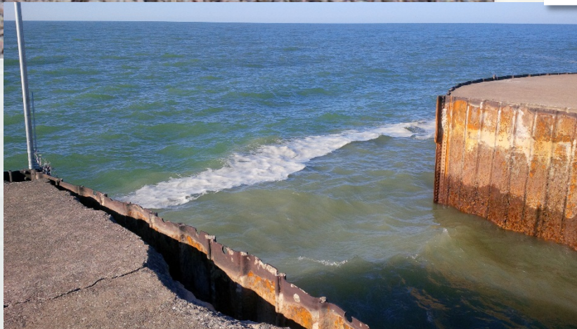
Barcelona – Complete Breach of Lakeside Structure
