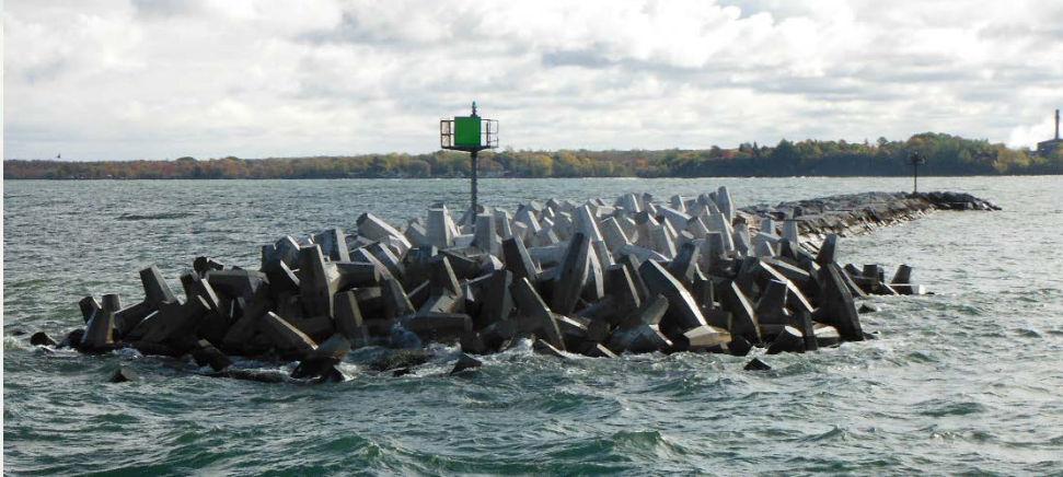
Finished Project with Dolosse at Western End
